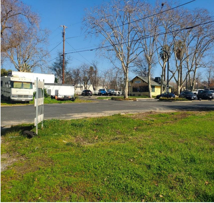
Photo 15: Near northeast corner, facing north. View of pole-mounted transformer on northeast adjacent property.
