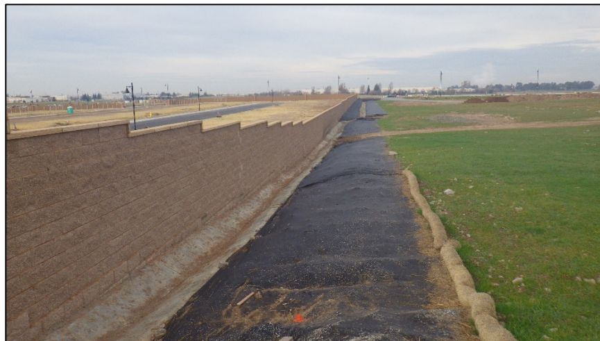
Photo 2: Looking west along the concrete lined v-ditch in the southern boundary of the Study Area.
