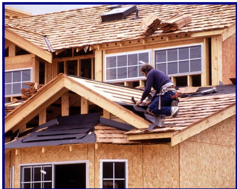
Rofer on a housing job site.
