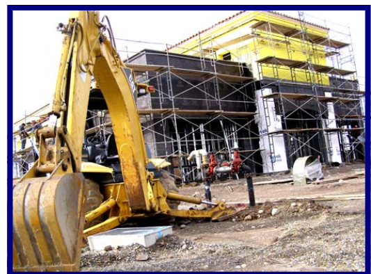
Construction of a business in Rocklin.
