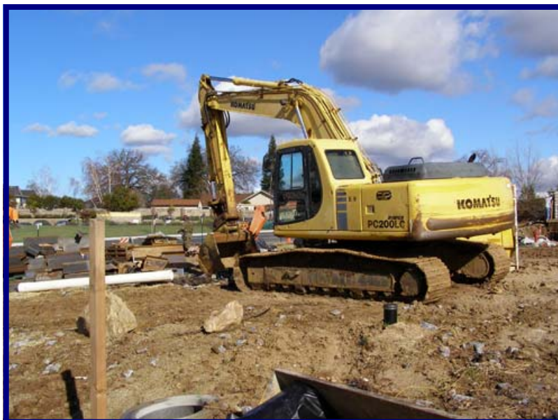
Preparation of a construction site.
