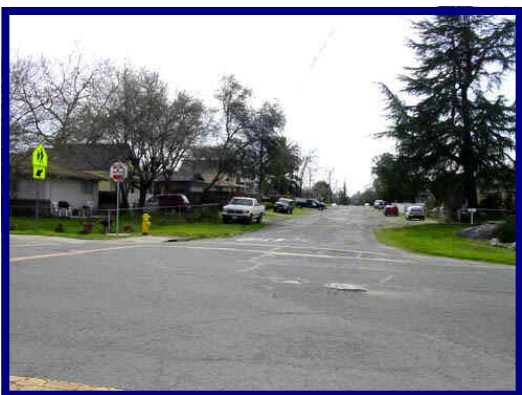
Safe Routes to School Project in Downtown Rocklin.
