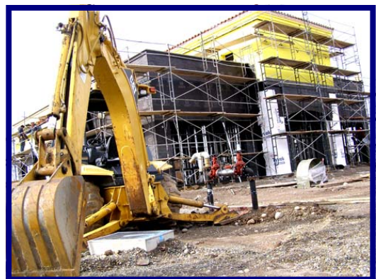
Construction of a business in Rocklin.
