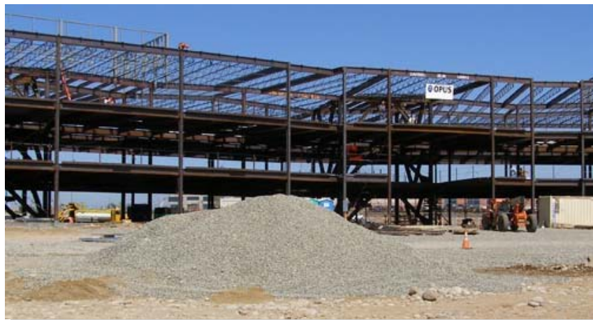
Construction of Opus West Corporation Class A offices on West Oaks Blvd., Rocklin
