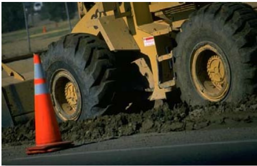
Construction of a new commercial/retail area
