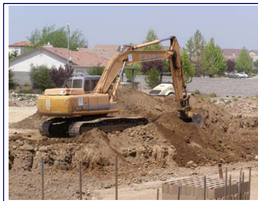
Construction of a new commercial/retail area
