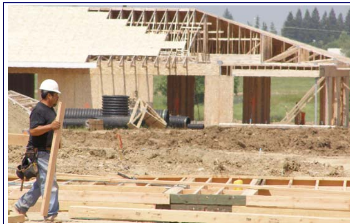
Construction of a residential area in Rocklin
