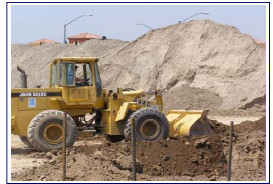
Construction of a new commercial/retail area
