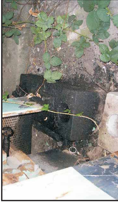
Photo 12: Stained soil beneath the oil gauge in the compressor room, north of the cutting shed. View to the east.
