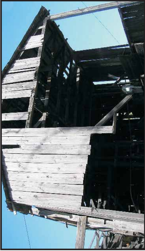
Photo 9: Cutting Shed dating back to the 1800s, north of the processing area. View to the west.
