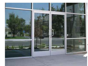
10'-0" HIGH CLEAR ANODIZED ALUM. STOREFRONT WITH MIRROR BLUE DUAL PANE GLASS.
