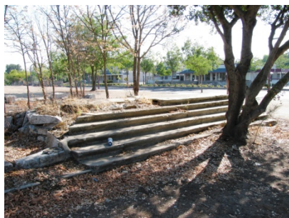
Remnants of steps from Rocklin's first school house and granite block foundation.
