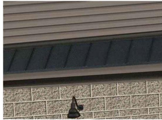
2 STANDING SEAM METAL ROOFING STANDING SEAM METAL ROOF AEP-SPAN, 12" SNAP SEAM COLOR: DARK BRONZE
