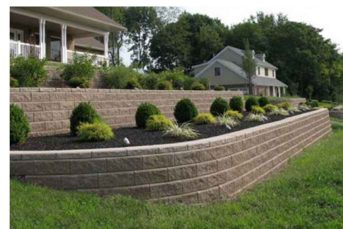
WALL TYPE "A" STACKED BLOCK RETAINING WALL EXAMPLE STYLE AND COLOR
