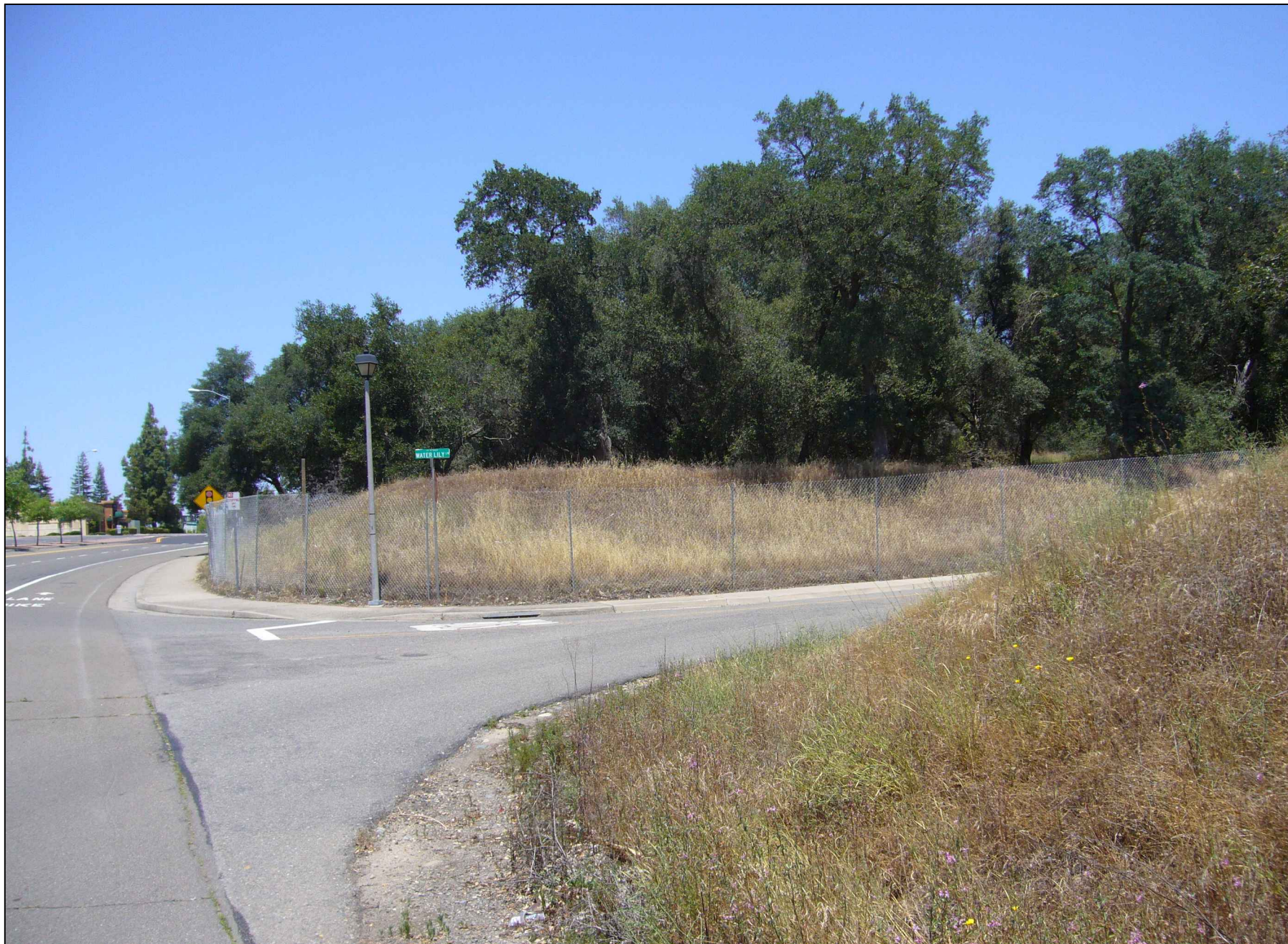
EXISTING - VIEW OF CORNER SIERRA COLLEGE BLVD. AND WATER LILY
