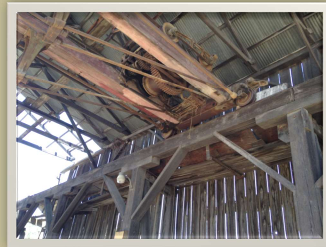
Salvaged gantry crane to be installed inside tap house
