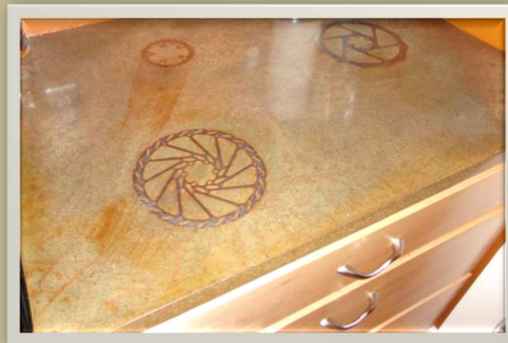
Concrete bar top with embedded artifacts
