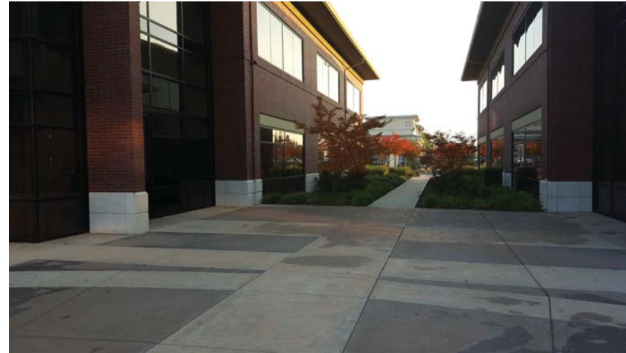
EXISTING WALKWAY BETWEEN 6554 + 6552 3
