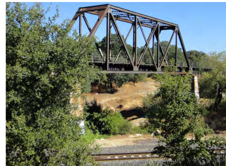
Nearby Rail Trestle Bridge
