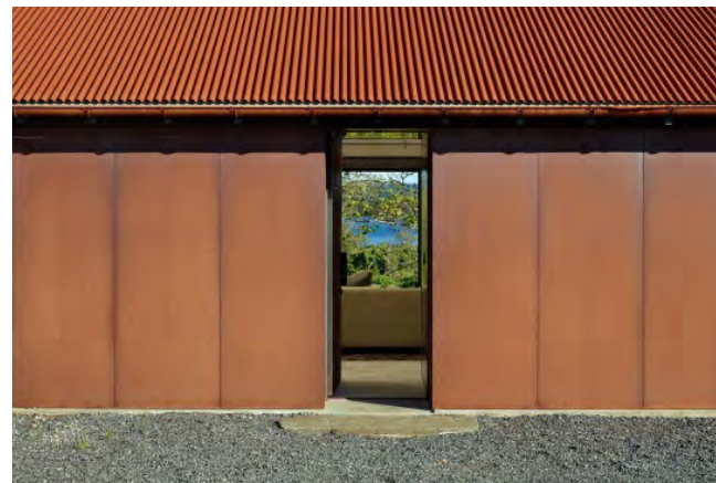
Weathered Steel Panels
