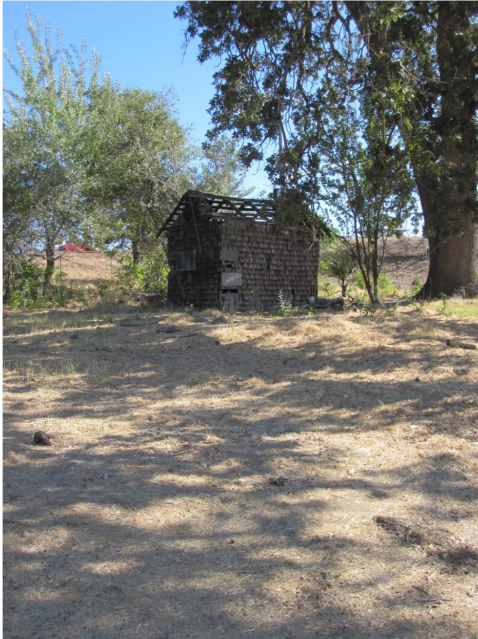
Photograph 2: Southwestern façades and surrounding area, view from the northeast.
