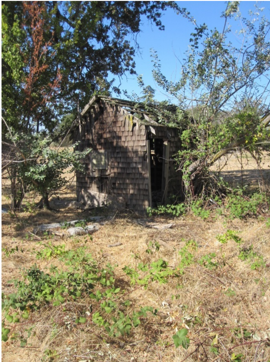
Photograph 3: Southwestern façades and surrounding area, view from the northeast.
