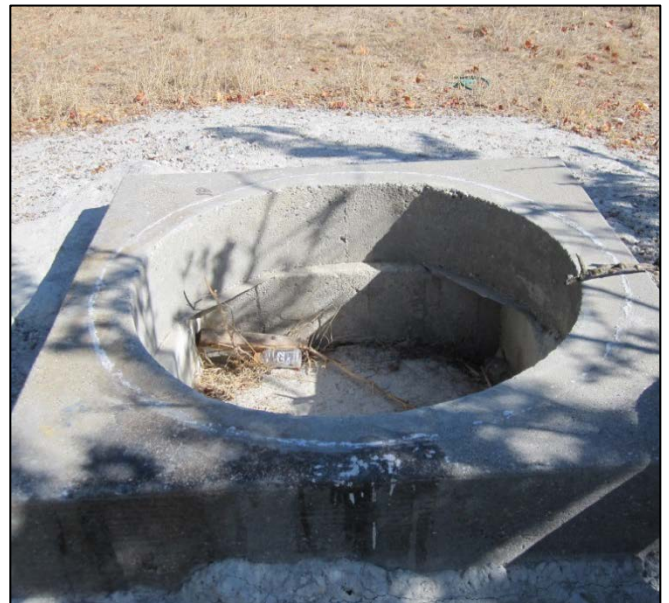
P5b. Photo 4770: Facing North, above view of well/cistern filled with modern concrete (Feature 2)
