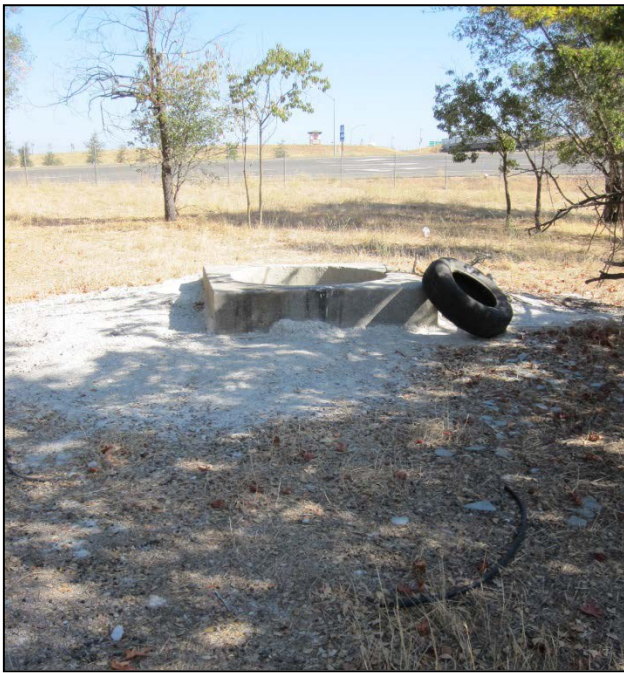
P5b. Photo 4769: Facing north, side view of well/cistern (Feature 2).
