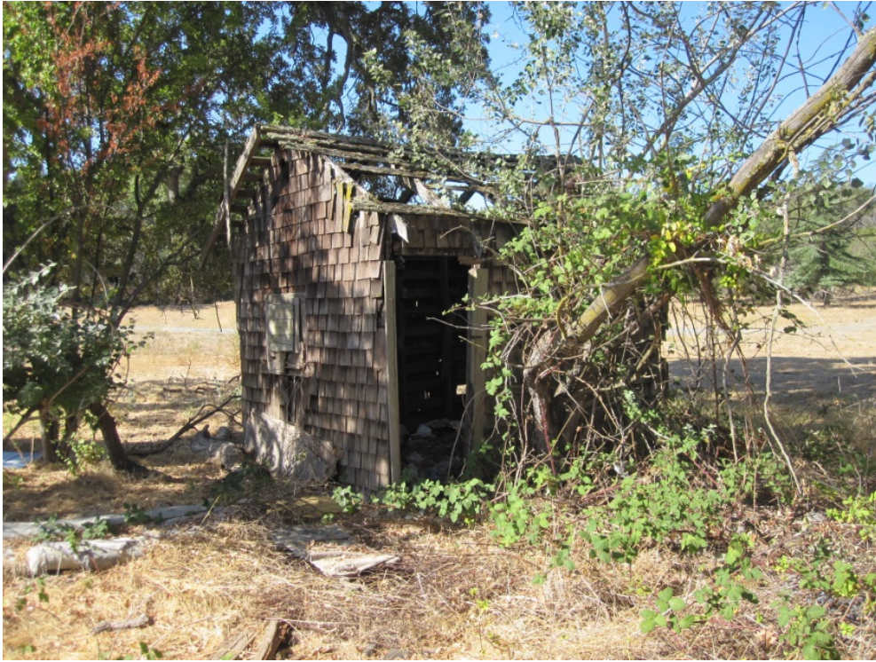
Photograph 1: Northeastern façades and entryway, view from the southwest.
