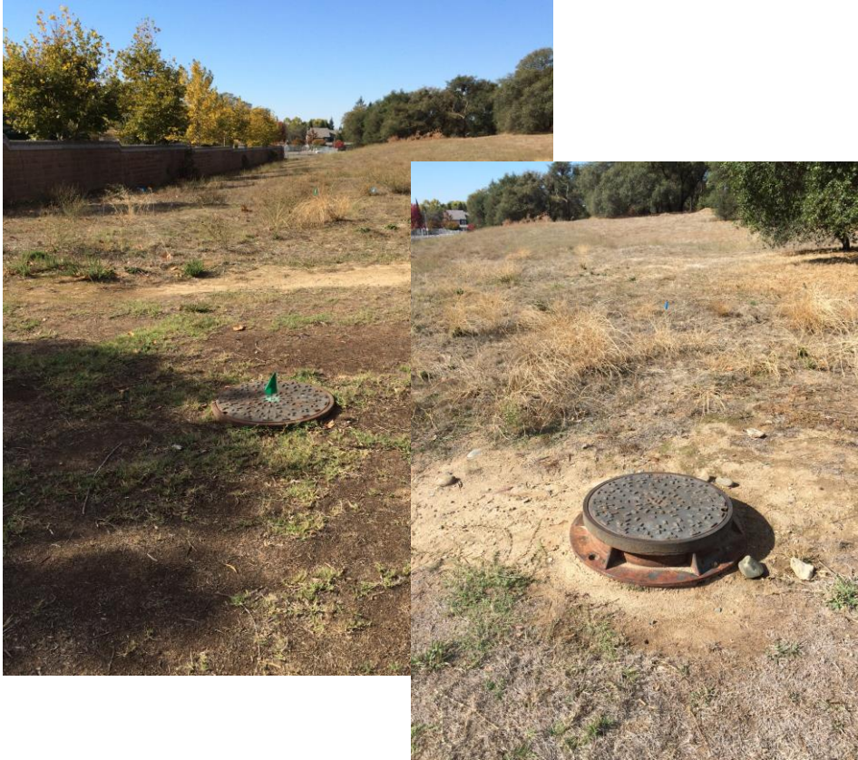
Photograph 13 - Two manholes located in the southeastern portion of the subject property.
