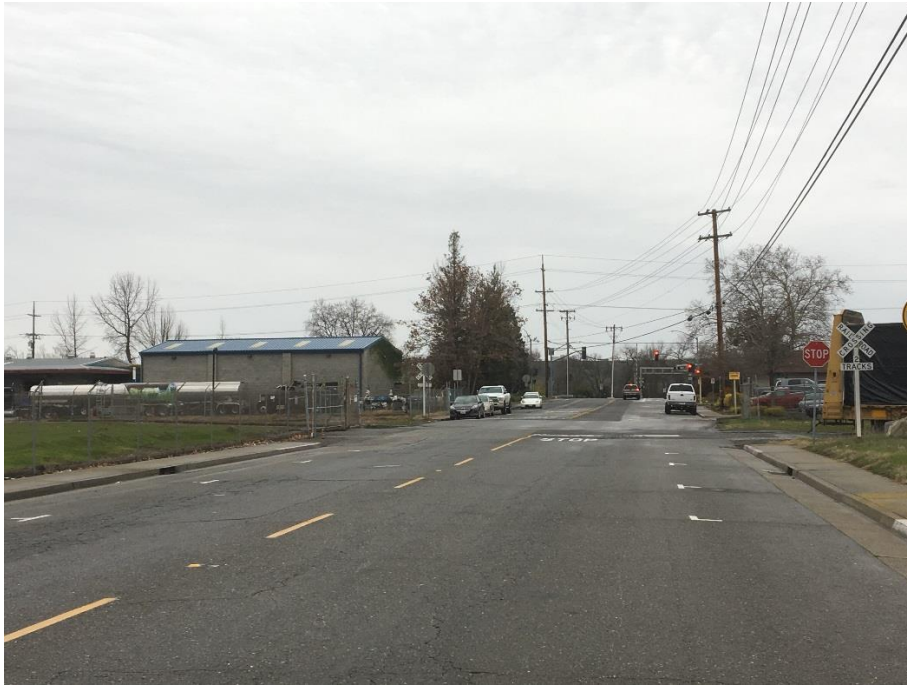
View of at-grade railroad crossing on Dominguez Road
