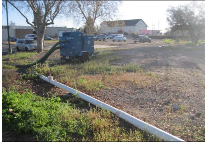
Photograph 3: Pump used to transport water from Quinn Quarry into the Rocklin Road Drainage System to the north of the Project Site.
