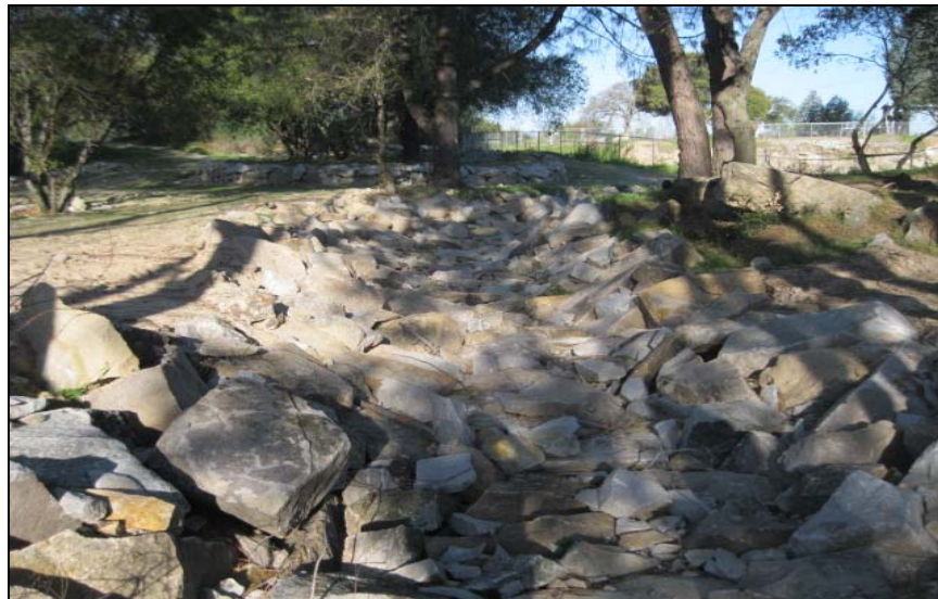
Photograph 4: View north of man-made ditch comprised of rip-rap.
