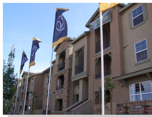
Vicara at Whitney Ranch attached homes.
