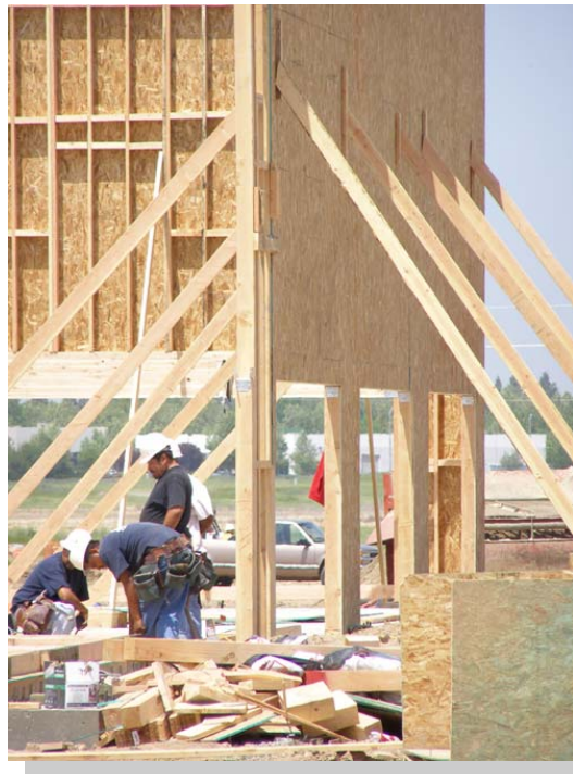
Construction of a new commercial/retail area.
