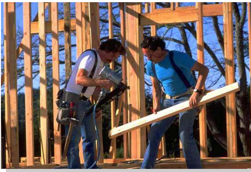
Building a structural frame.
