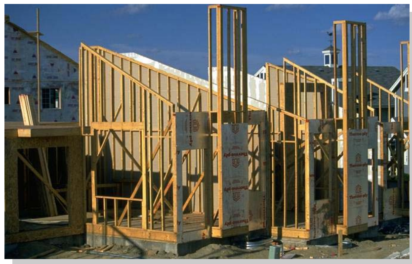
Residential home construction.
