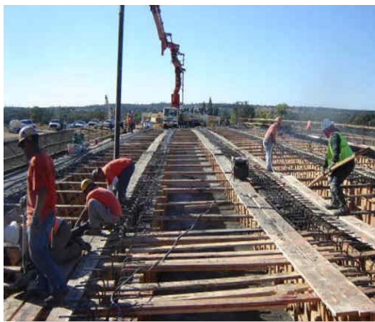
Construction of Sierra College Blvd/I-80 Interchange
