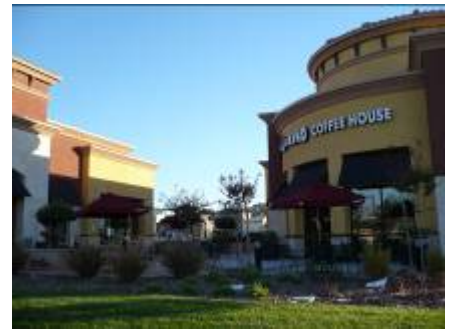
ACCEPTABLE Mansard roof wraps around entire building.
