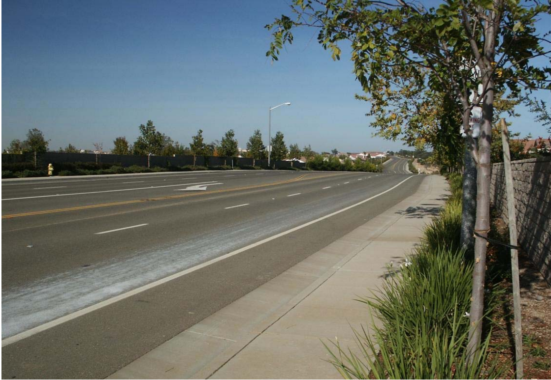
Figure 3.4-2. Narrow City-maintained shoulder plantings along Park Drive near Lake Tahoe Ct. No center median plantings are present in this area.
