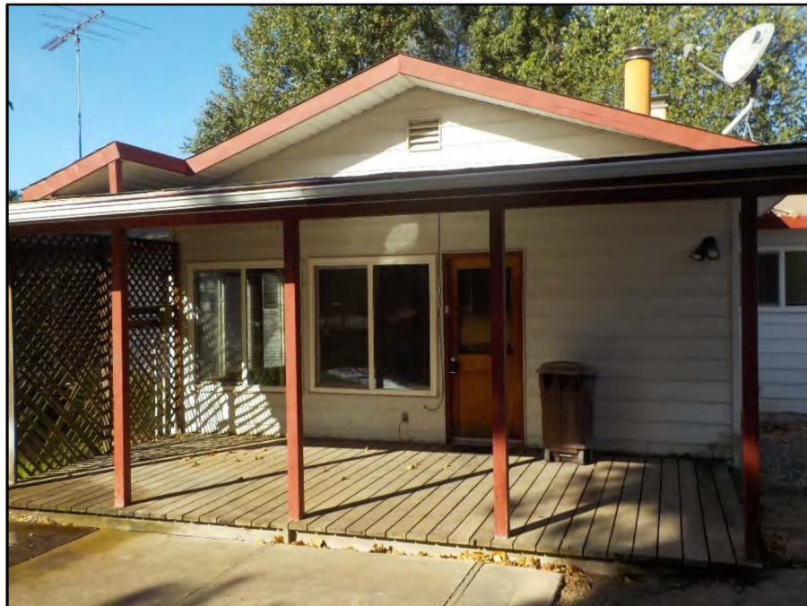
Eastern facing façade of residence (view west; September 25, 2020).
