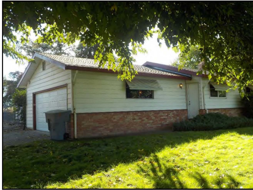
Attached garage residence, northwestern façade (view southeast; September 25, 2020).
