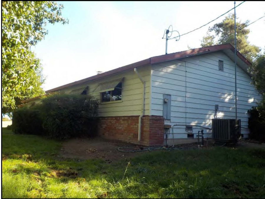
Western facing façade of residence (view northeast; September 25, 2020).
