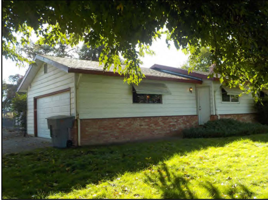
Figure 4. Attached garage at residence, northwestern façade (view southeast; September 25, 2020).
