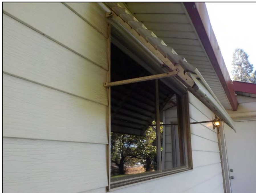
Window detail, western façade (view south; September 25, 2020).
