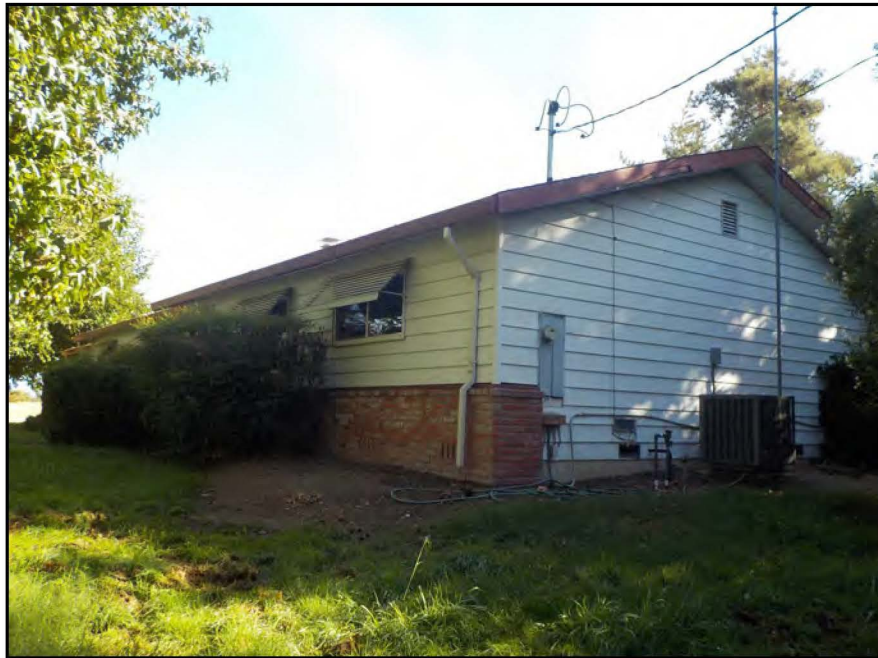
Figure 5. Western facing façade of residence (view northeast; September 25, 2020).
