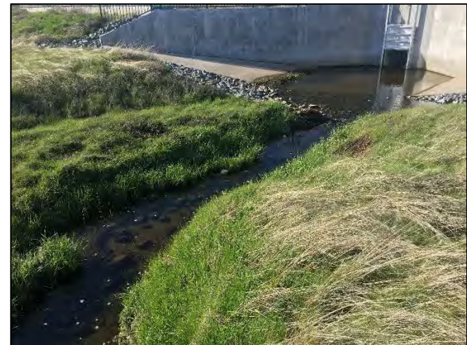
Photo 32. Culvert in Orchard Creek (OC).
