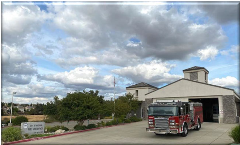
Station 25, 2001 Wildcat Boulevard
