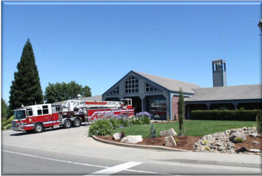
Station 24, 3401 Crest Drive
