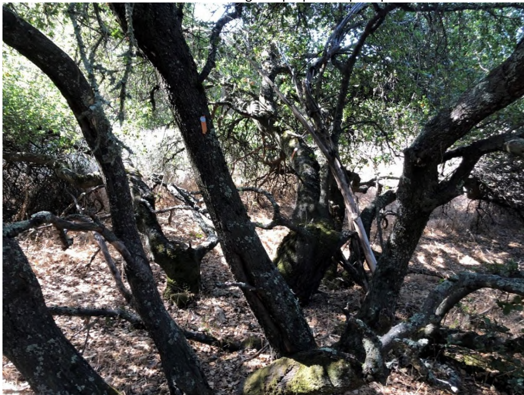
Photo 12: Typical, note basal defects, excessive dead wood, and poor structure.
