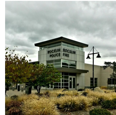
Rocklin Police & Fire Facility
