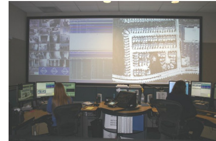
Rocklin Emergency Communications Center
