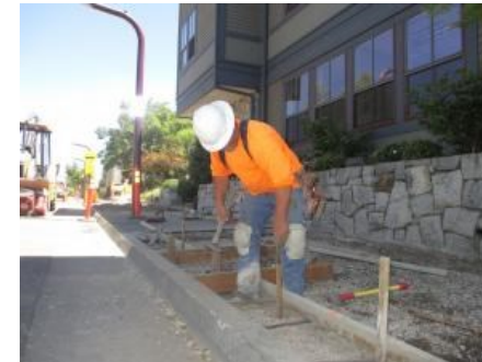
Sidewalk Repair on Rocklin Rd.
